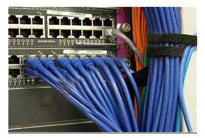
Switches are a special type of hub that offers an additional layer of intelligence to basic, physical-layer repeater hubs. A switch must be able to read the MAC address of each frame it receives. This information allows switches to repeat incoming data frames only to the computer or computers to which a frame is addressed. This speeds up the network and reduces congestion.
